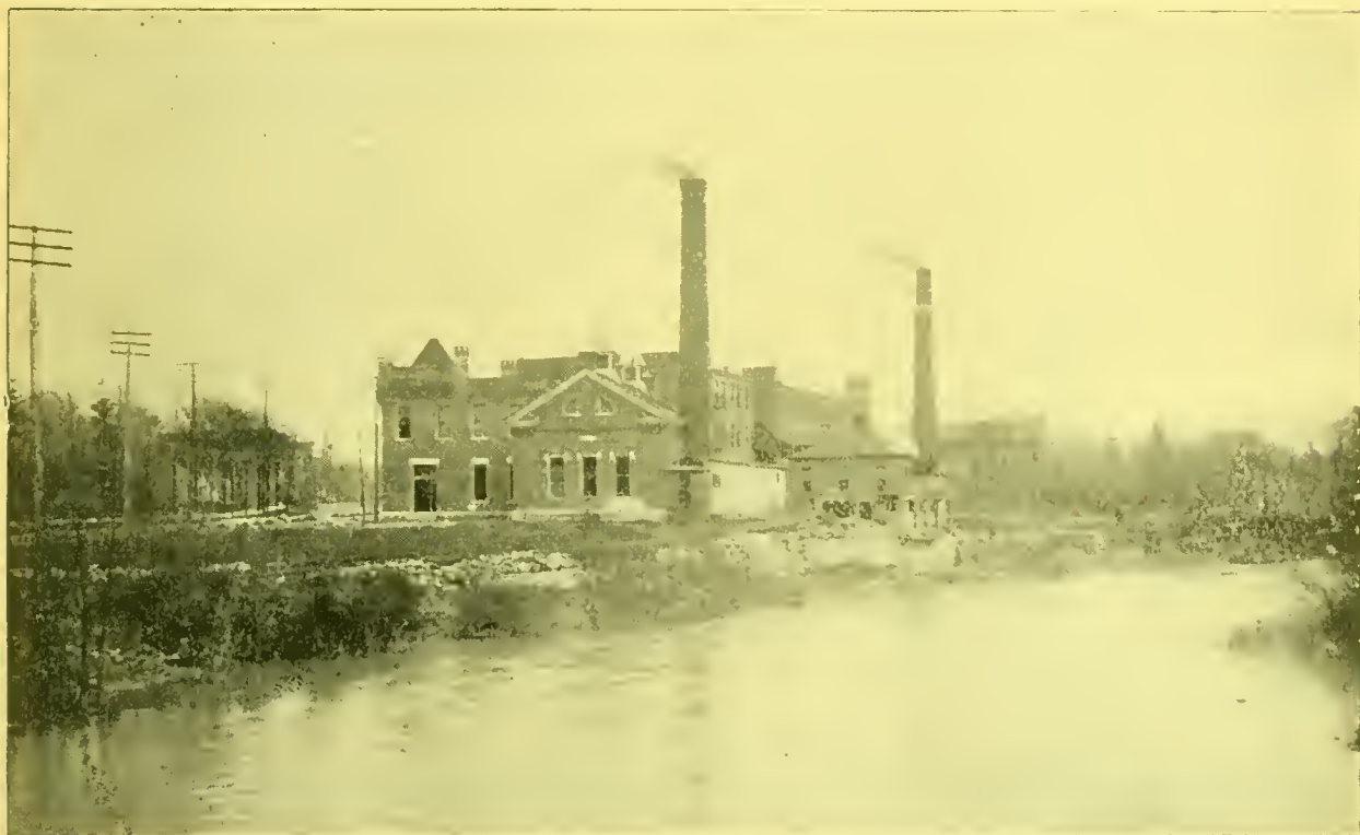
THE BRISBANE CURVE FROM TONAWANDA BRIDGE.
